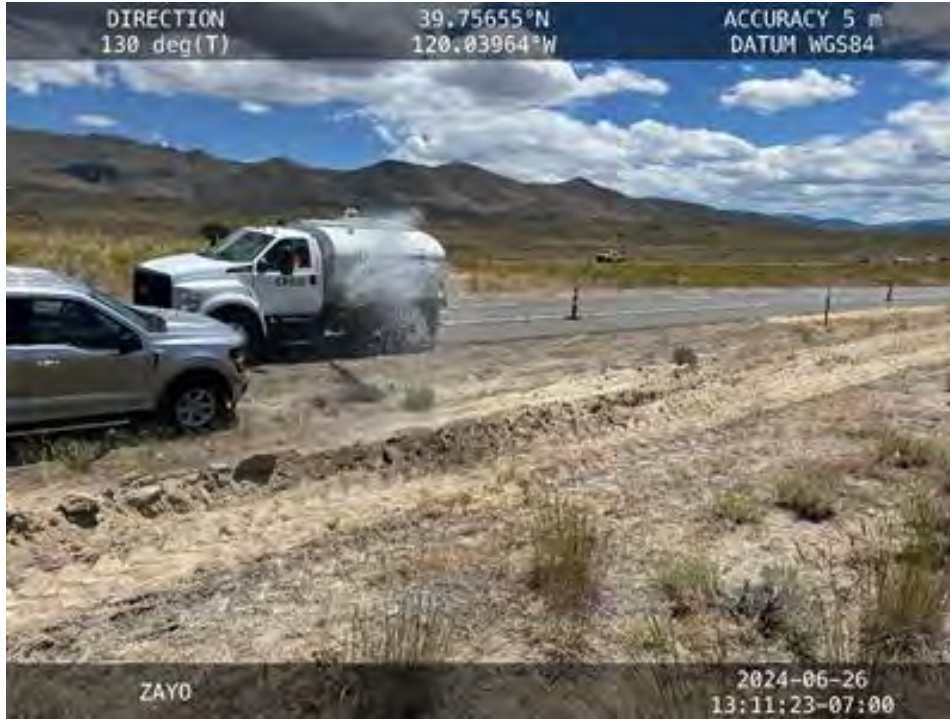
Figure 8. View of water being used for dust mitigation (Lassen County).
