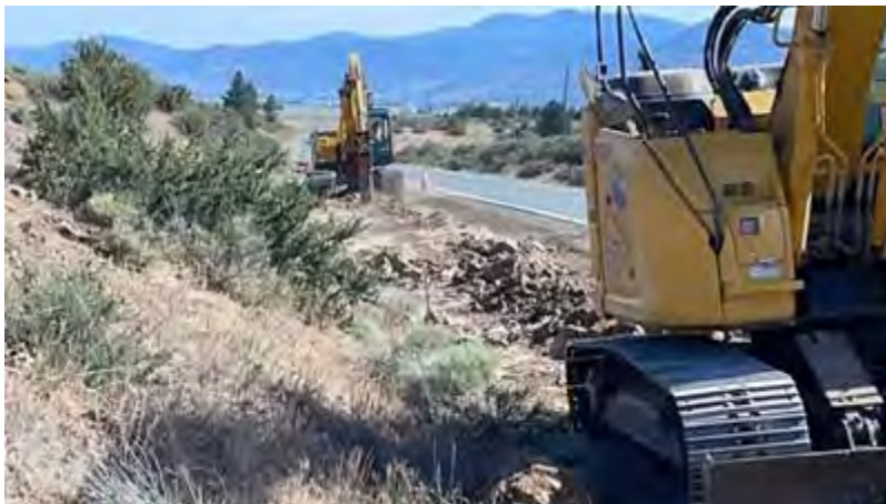
Figure 15. Overview rock hammer progress facing northeast.
