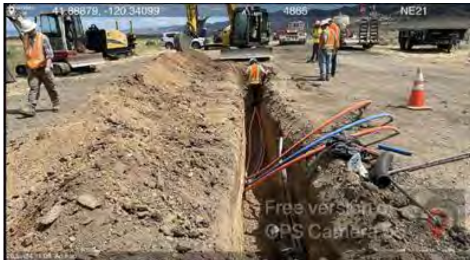
Figure 7. View of tie-in operations.
