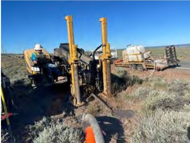
Figure 12. HDD overview facing southwest.
