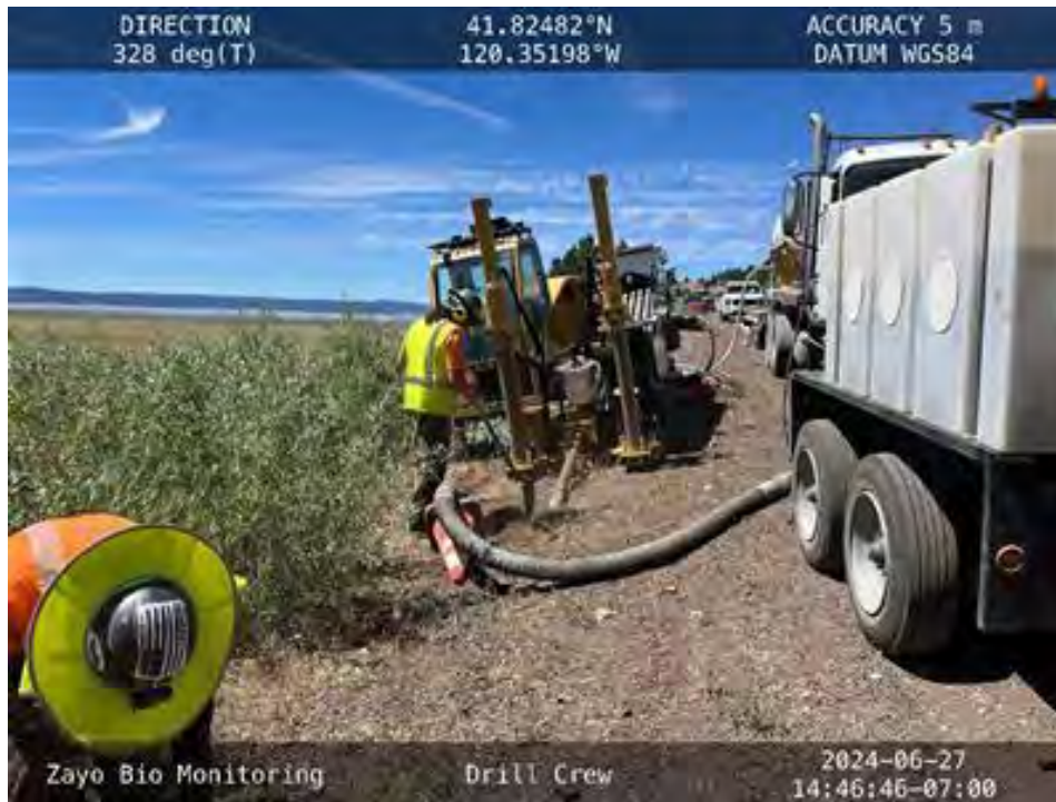
Figure 2. View to the north of drilling crew in Modoc County.
