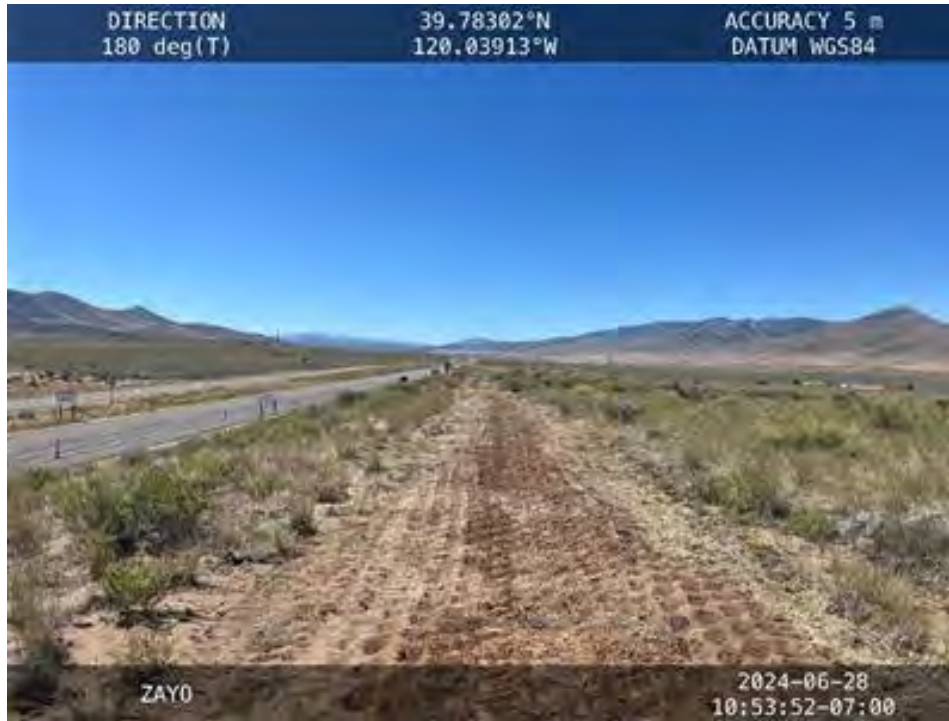
Figure 6. View to the south of the graded and compacted plow line along the RL (Lassen County).
