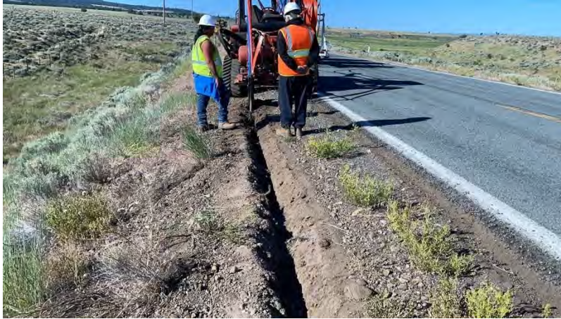
Figure 14. Overview plow monitoring facing south.
